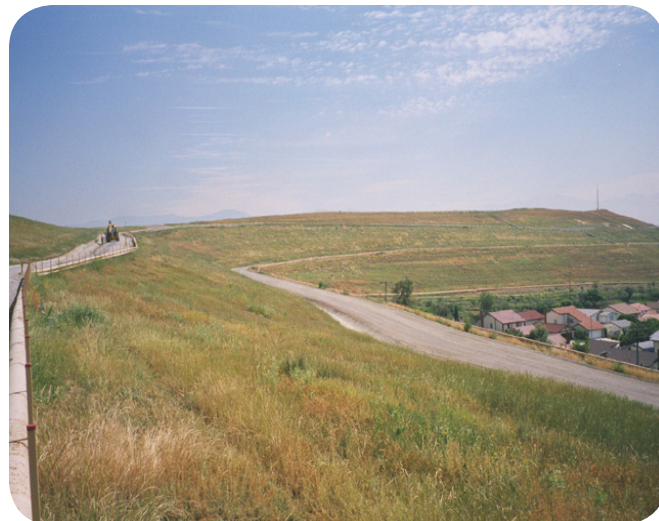
Example of ET cover used at Operating Industries, Inc. Landfill Superfund site.
