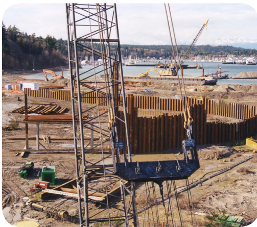
Installation of sheet piling
