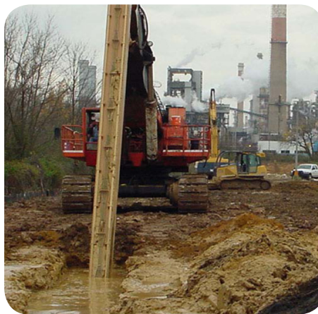
Excavation of a slurry wall trench
