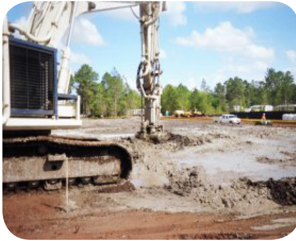
Large augers inject and mix binding agent with contaminated soil.
