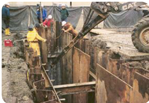
Construction of a PRB in Sunnyvale, CA
